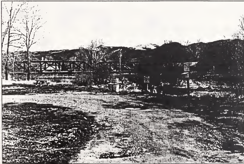
Looking Northeast at Bridge near Boat Ramp
